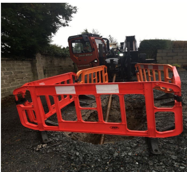
Marian Park Drilling for Pipe Installation
