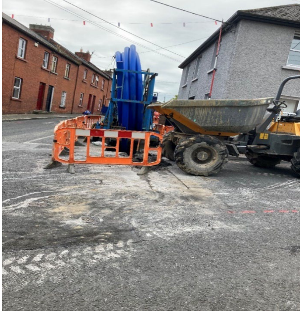
Installation of pipe by Directional Drilling
