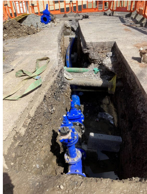
Installation of pipe by excavation
