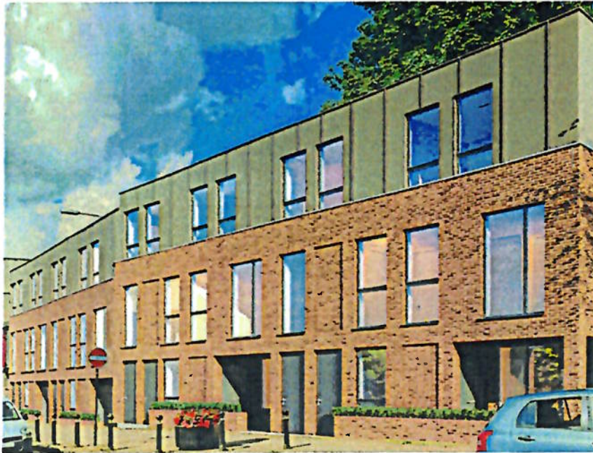
20 Units at St. Brigid's Terrace, Cavan – currently under construction.
