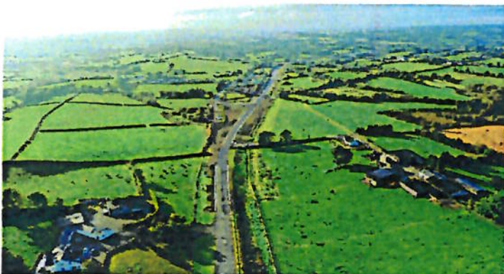
Aerial view southward of the realigned Mainline at the northern tie-in in the townlands of Drumhawragh & Ballytrust.
