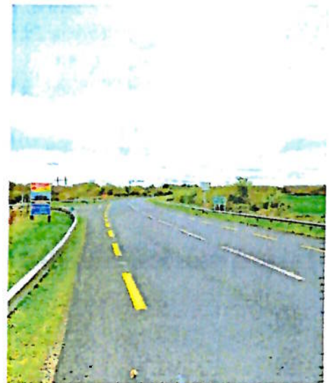
Above: Completed EWS Works N55 Pottahee
