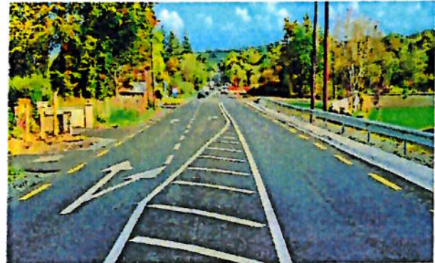
Above : New right turning lanes for southbound traffic turning into the L2508 Caughoo and northbound traffic turning into the L6568 Kilmainham.
