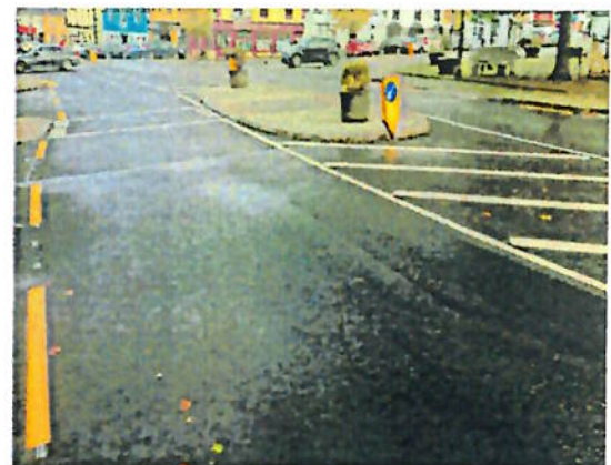
Above: L3503 Carrickallen – Improved Road Surface, Road Markings, High Friction Surfacing and Signage
