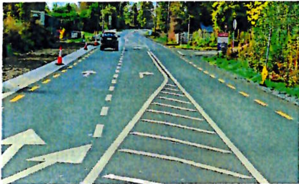
Above : New right turning lanes for southbound traffic turning into the L2508 Caughoo and northbound traffic turning into the L6568 Kilmainham.
