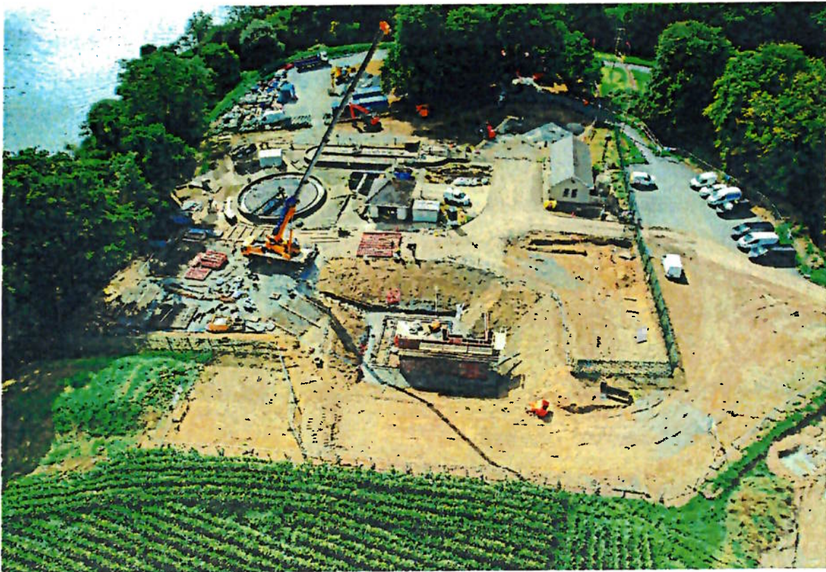
Progress to date on site Upgraded Virginia Wastewater Treatment Plant
