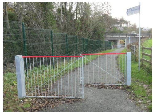
Figure 10: staggered gates prevent unauthorised vehicular access. The gates can be opened on request for events with large footfalls
