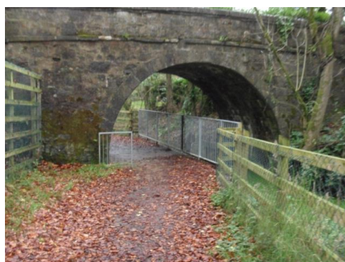
Figure 4: a simple railing pushes users out from the low side of the arch. Railings and fencing prevent any watery mishaps!
