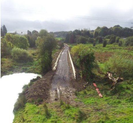
Figure 11: View of Monaghan greenway under construction.
