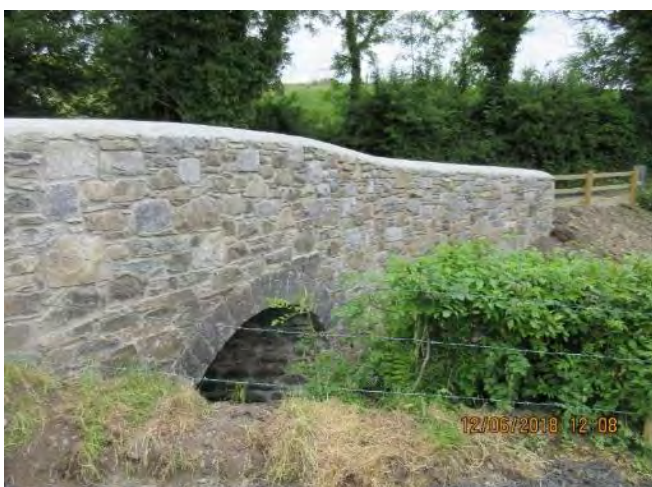
Burnew Bridge Before and After
