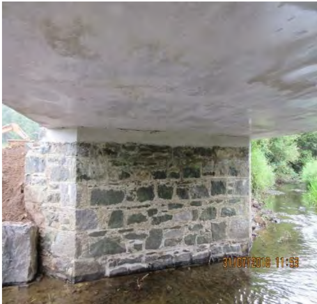
Drumfomina Bridge - Before and After
