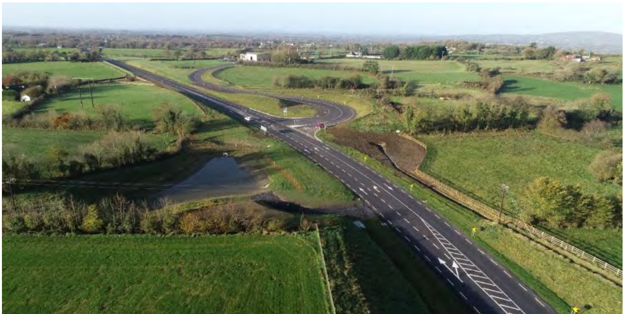
Aerial picture of surfacing and lining on Phase 1 at Garrymore
