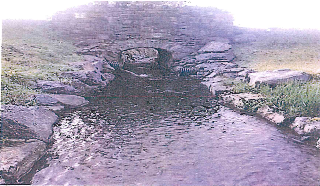
Lackenmore Bridge, Ballyjamesduff – post repair.
