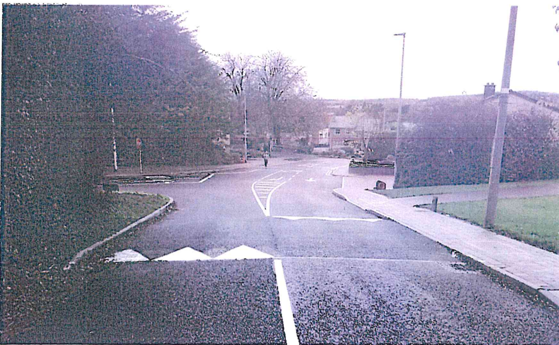
New layout at St. Clare's Junction, Cavan Town
