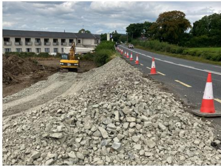
Embankment and road repair on N3 at Lakeside Manor Virginia.
