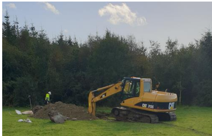
Right: Excavation of a Trial Pit
