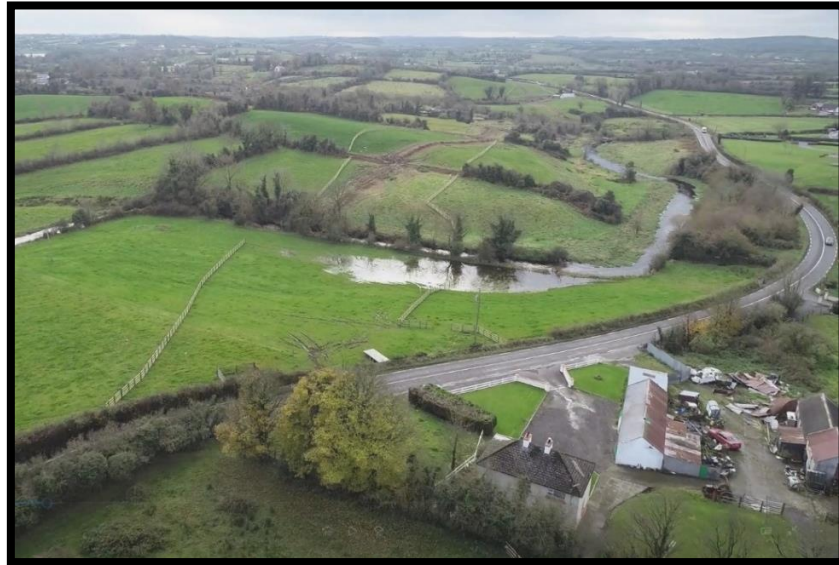
Aerial view of the boundary fencing of the route of the proposed road alignment, close to the existing N55 alignment at Ballytrust lower and Legwee.
