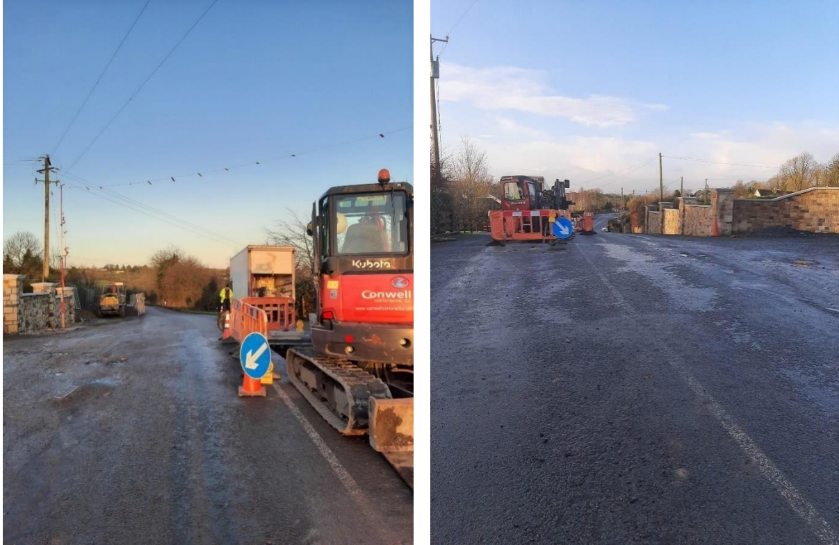
Works on Shankill – Billis Mains Rehab Project in progress
