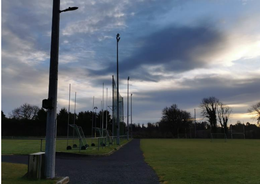
Ballymachugh GAA- upgrade of lighting to LED Lighting
