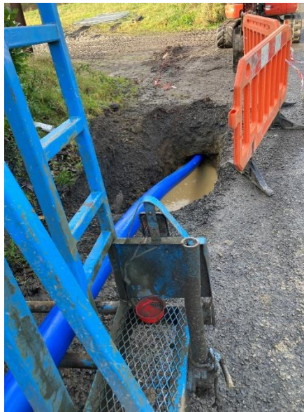
125mm HDPE pipe installation by directional drilling at Shankill Billis
