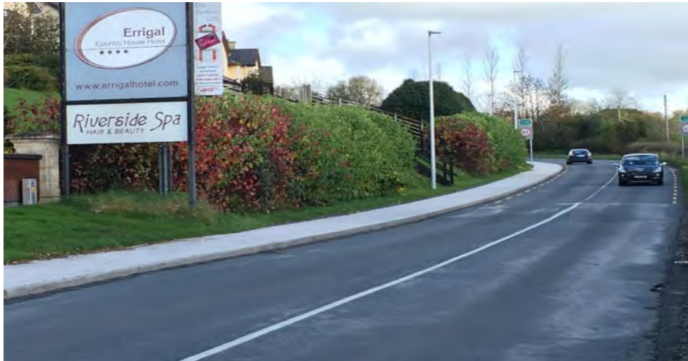
Footpath & Public Lighting on R188 approach to Cootehill
