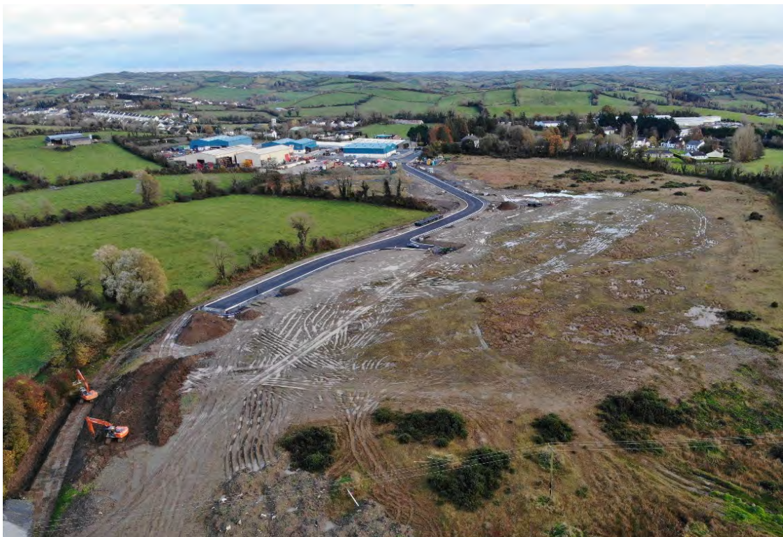
Cootehill Enterprise Park under construction
