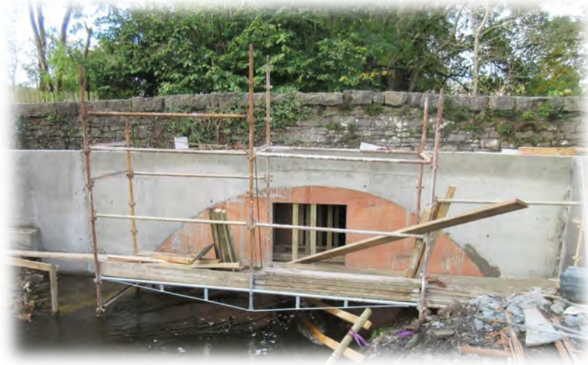
Drumlark Bridge – Widening of narrow bridge to accommodate new footpath
