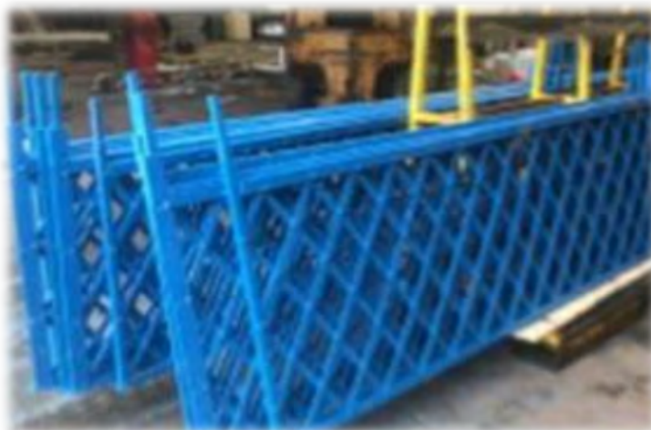
Above: Recently refurbished railings
