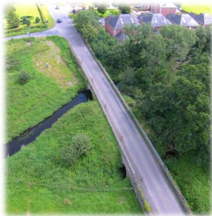
Dunancory Bridge with restricted carriageway width prior to works.
