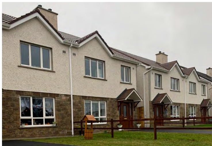
New Housing at Ashgrove, Ballyjamesduff
