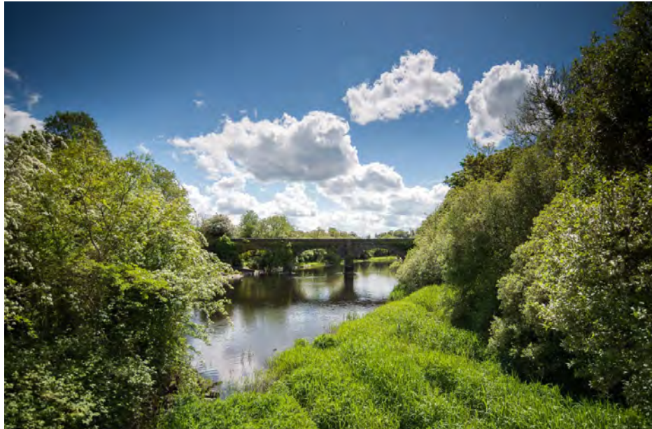
Belturbet Railway bridge over the river Erne.
