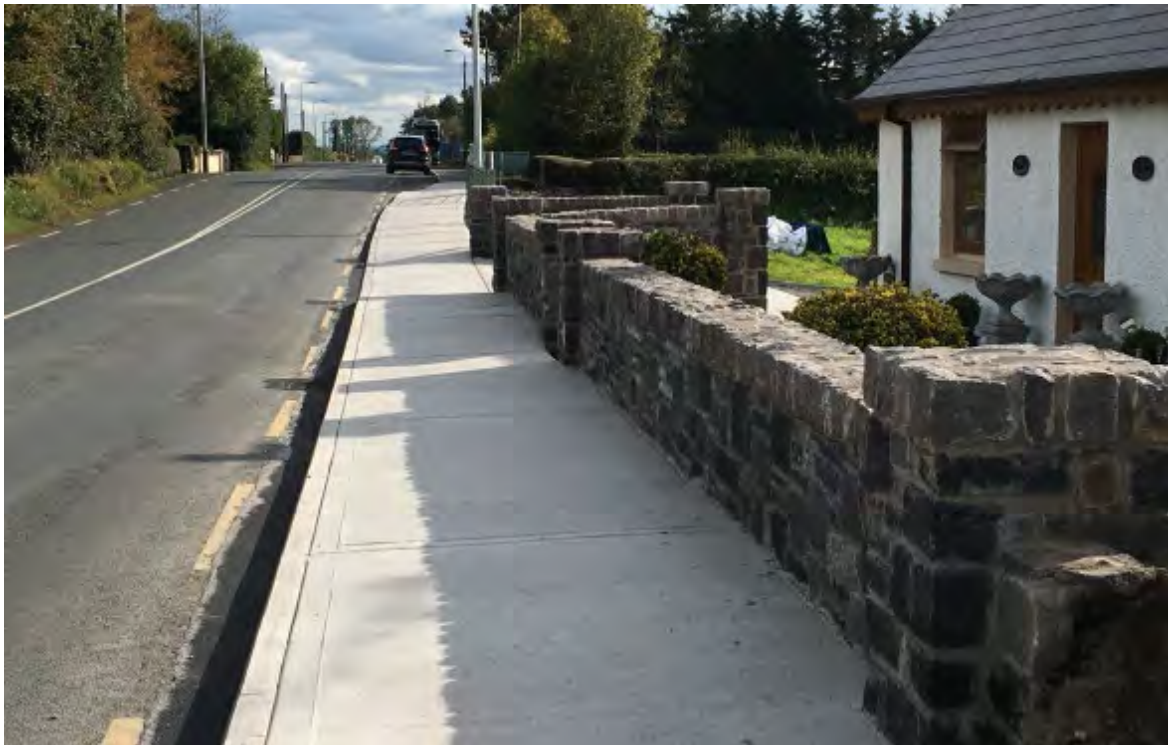
Footpath & Public Lighting on L3013 in Ballyjamesduff
