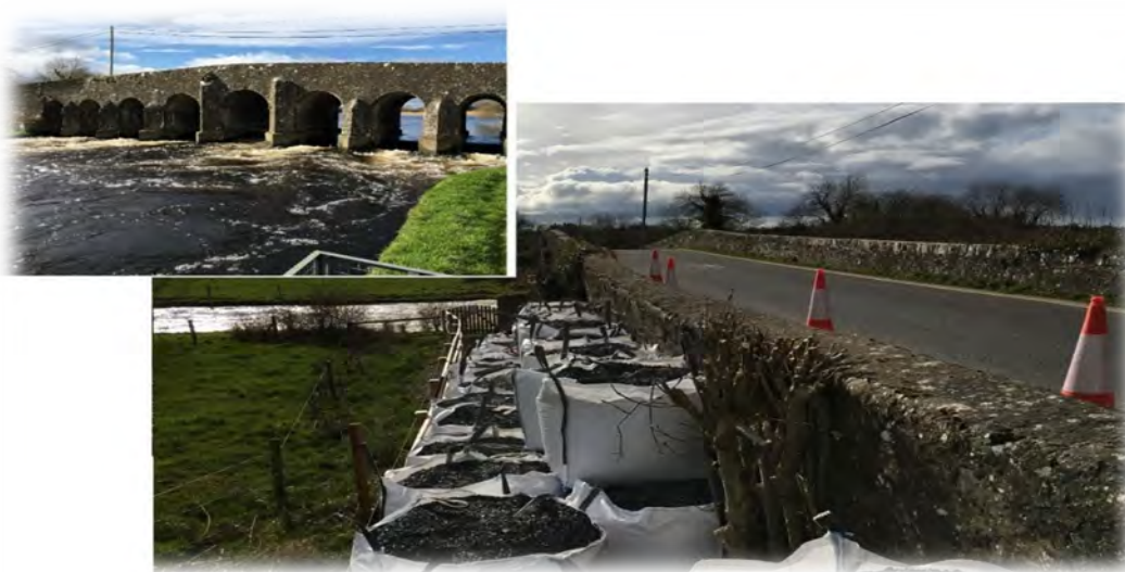
Above: L3024 Nine Eyed Bridge at Stramatt
