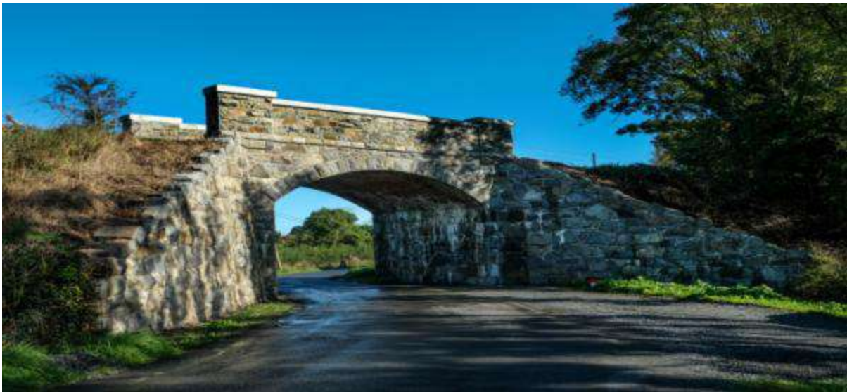
Crossdoney Bridge, Crossdoney.
