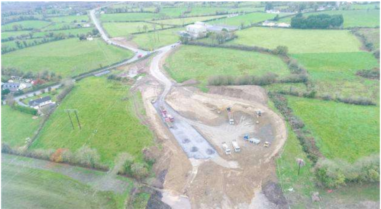
Aerial picture of excavation works on Phase 1 at Garrymore
