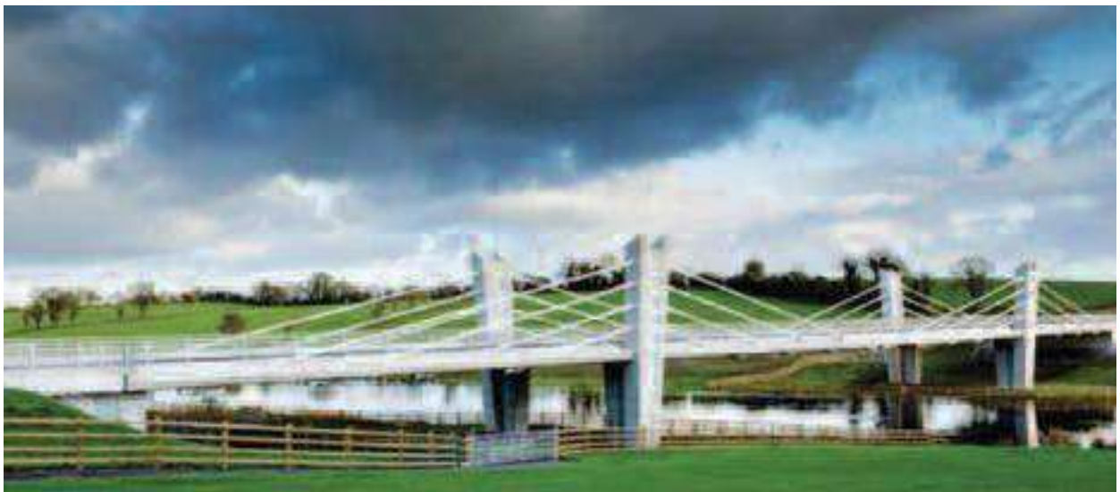
Extradosed Type Bridge over the River Erne
