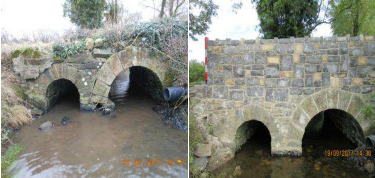
Keadew Bridge - Before and After
