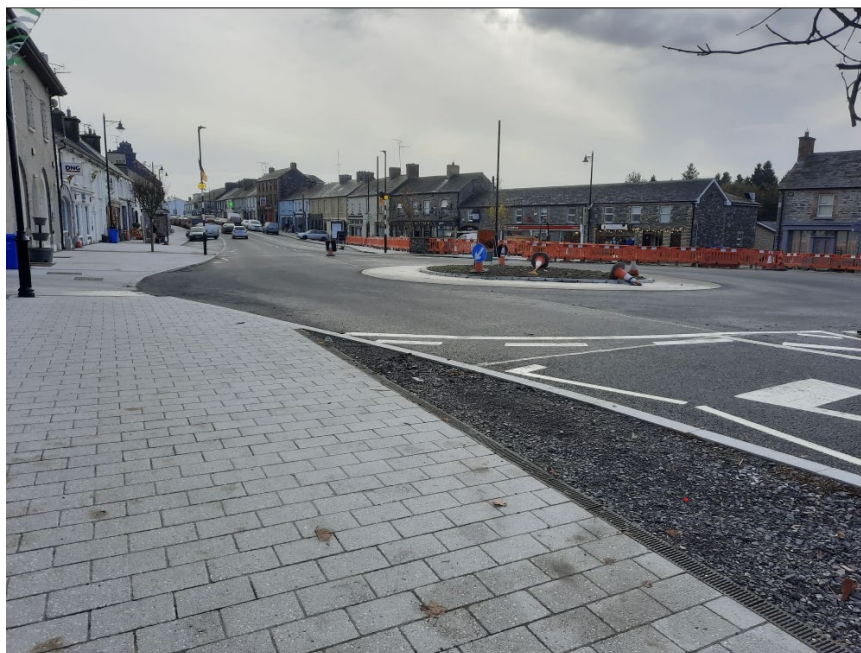
New Roundabout at Junction of N3 and Ballyjamesduff Road in Virginia.
