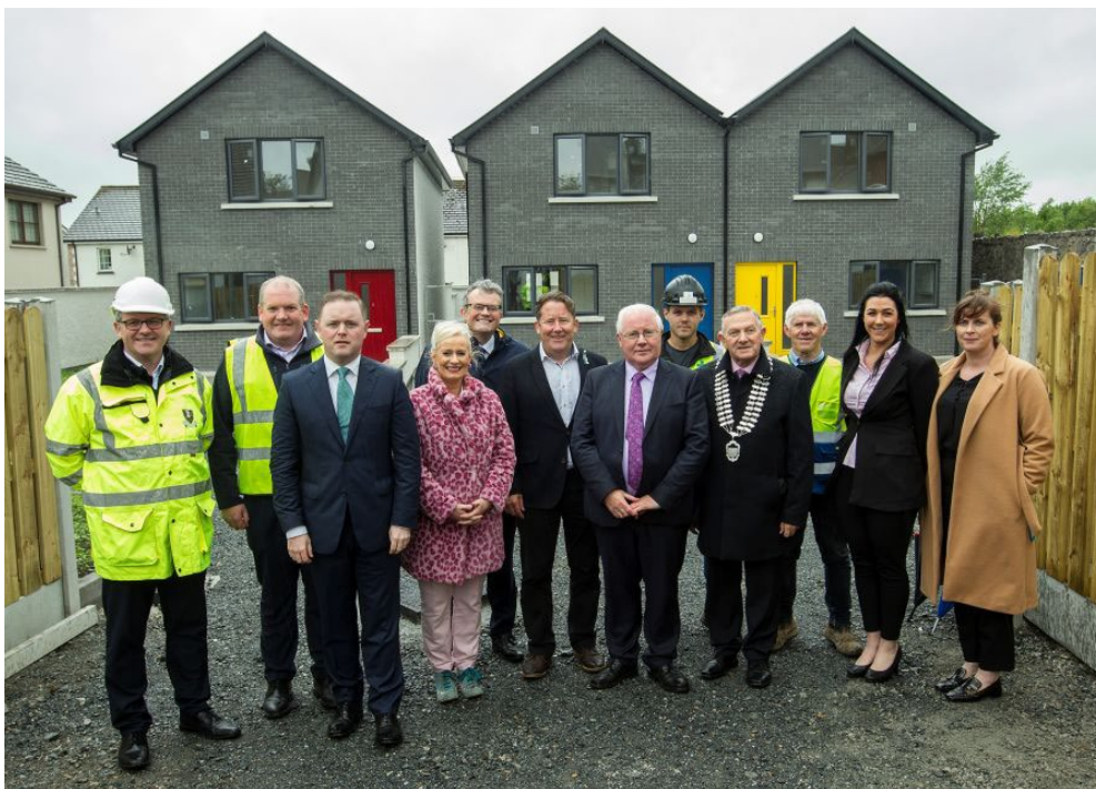
On 26 May 2022, Minister O'Brien inspected progress on the construction of six new social houses by local contractor Crosserlough Construction in Butlersbridge.
