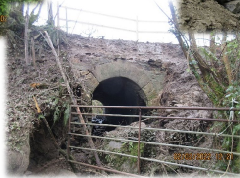
Cullentragh Bridge R188 (Before Devegetation, After Devegetation & After Rehabilitation Works)
