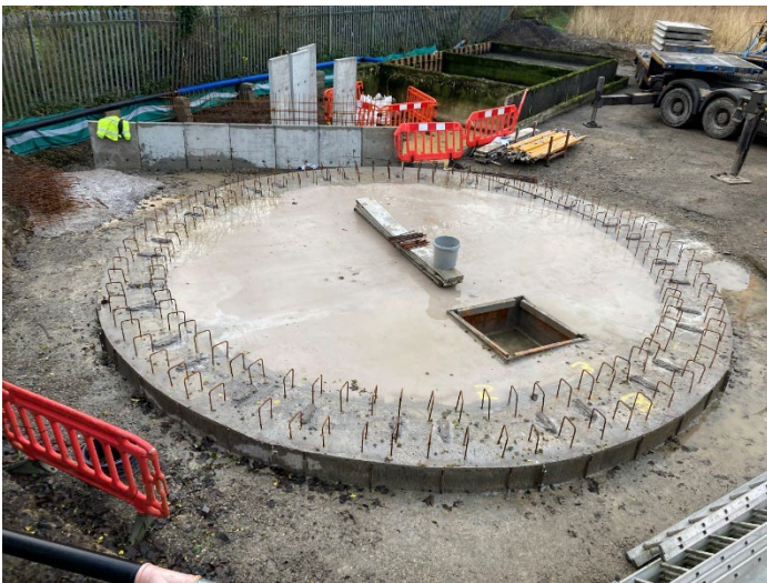
Base for New Storm Tank
