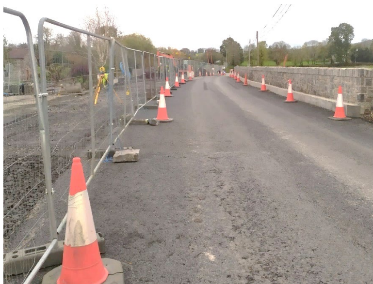
Derrylea Bridge Widening Works
