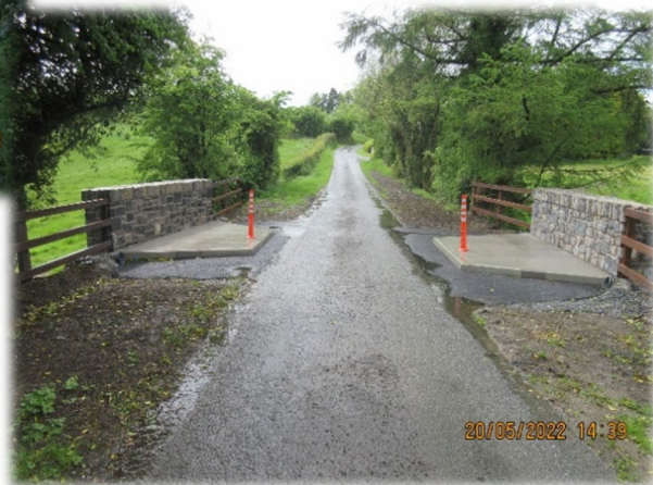
Moher Bridge L7504 (Before Rehabilitation Works & After Rehabilitation Works)
