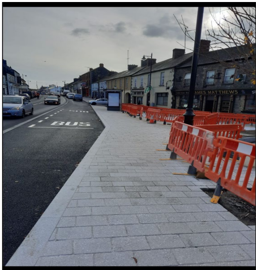
New footpath paving and Bus Stop
