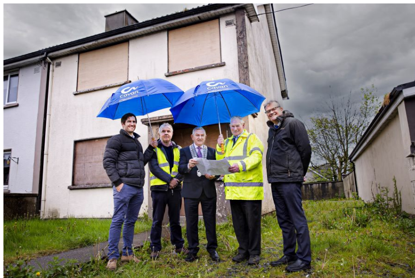
Pictured surveying ongoing renovation and deep energy retrofit work at a vacant social housing unit at John Paul Avenue, Tullacmongan, Cavan are (from left)
