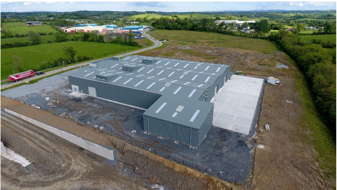
Cootehill Enterprise Park – Construction of PQE Building June 2022
