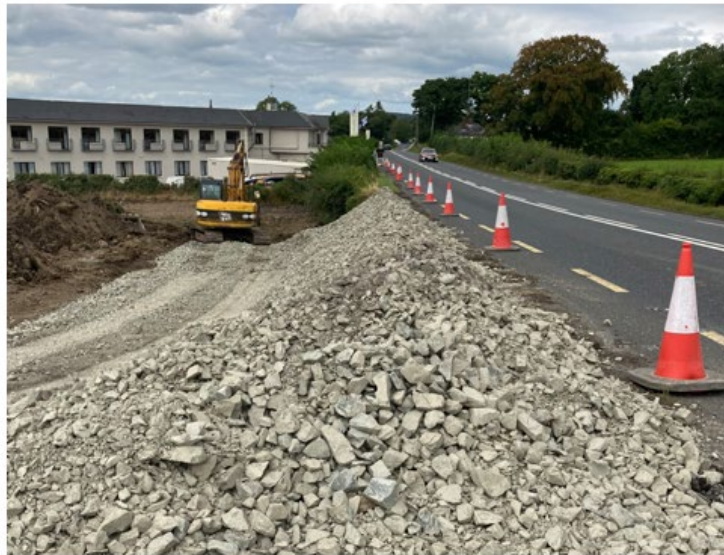
Embankment and road repair on N3 at Lakeside Manor Virginia.
