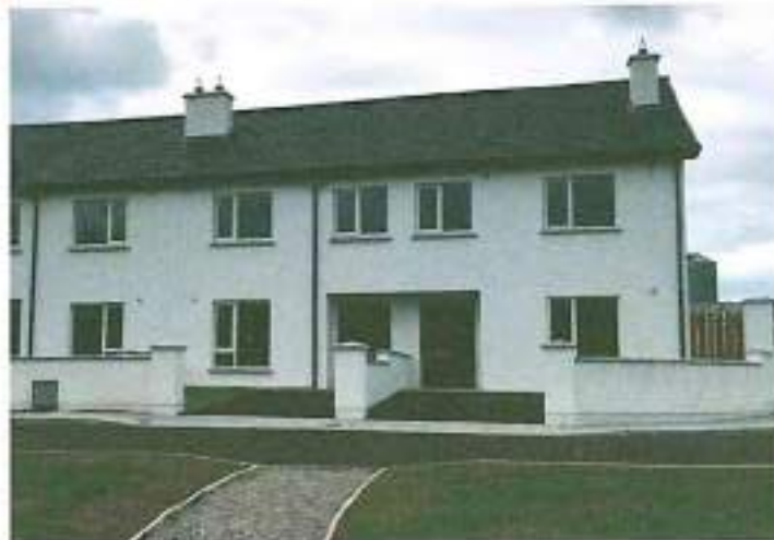
New Housing Scheme in Butlersbridge completed in 2018.
