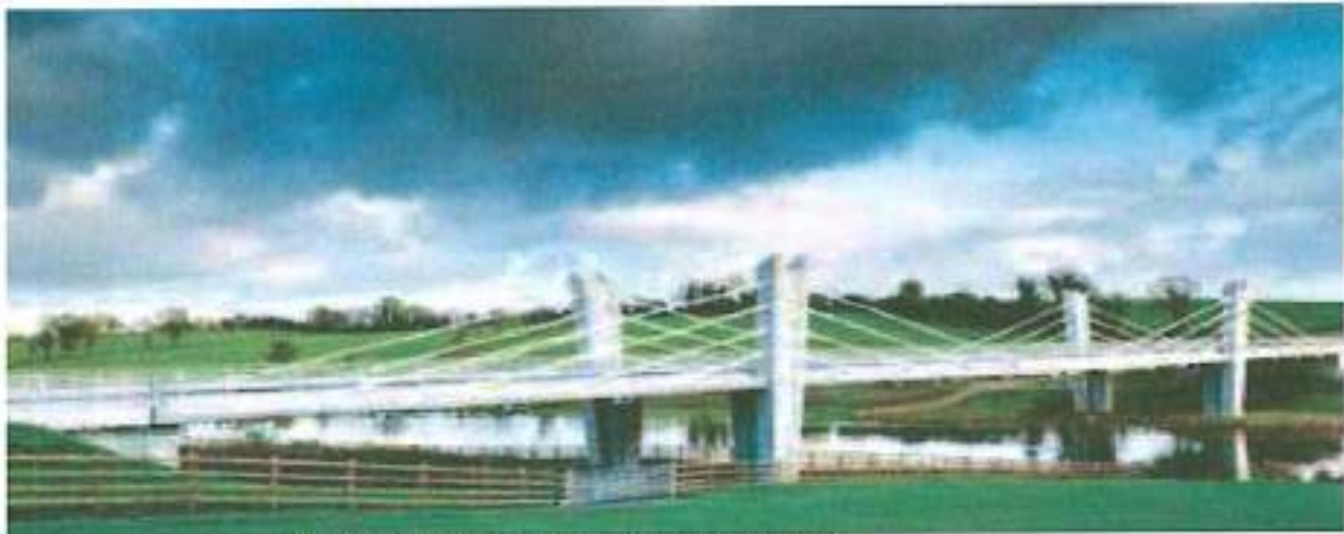
Extradosed Type Bridge over the River Erne
