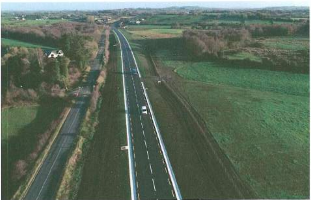
Aerial picture of new alignment works on Phase 2 at Oghill
