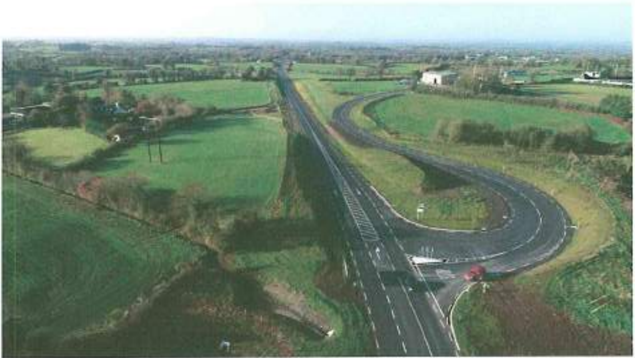
Aerial picture of new alignment works on Phase 1 at Garrymore
