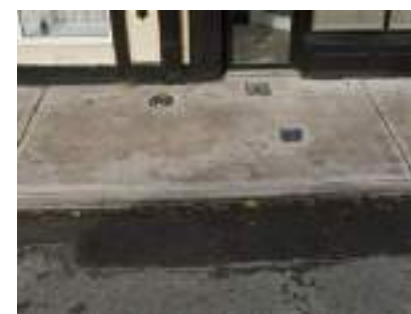
Figure 90 - Pavement at Barrack Street
