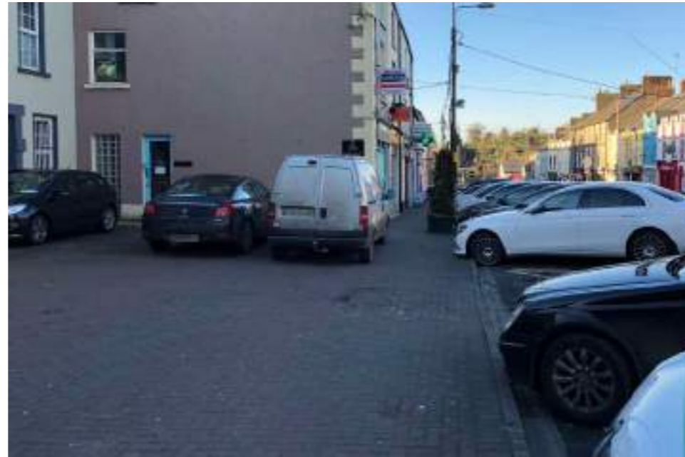
Bailieborough - existing: uneven paving littered with chewing gum and current design enables parked cars to overlap the kerb.
