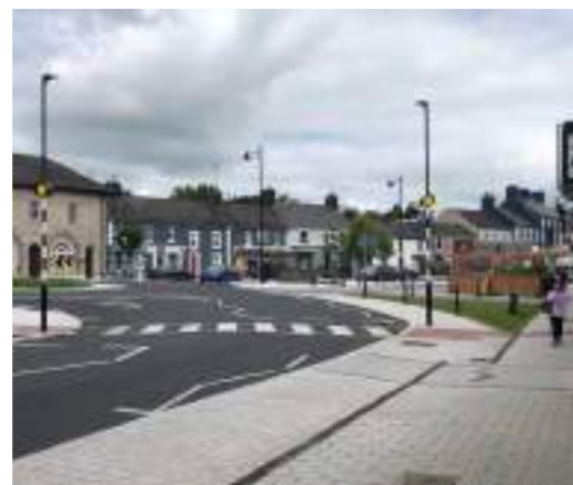
Figure 83 -Virginia Public Realm - Recently Completed by Cavan County Council
