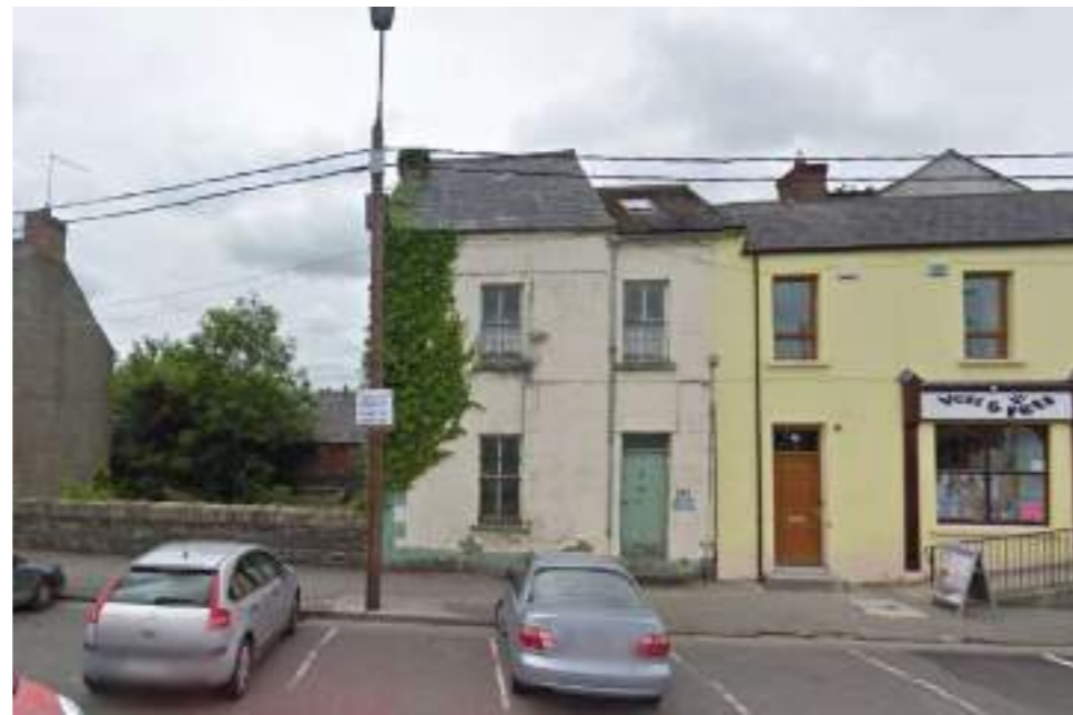
Bailieborough - existing: key façades in need of refreshment
