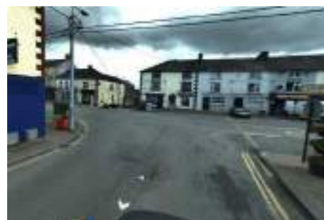
Figure 108 - Existing Junction View
