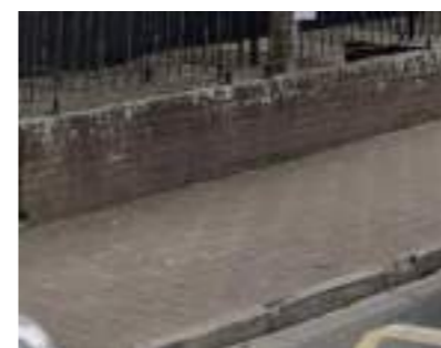
Figure 93 - Pavement at Main Street
