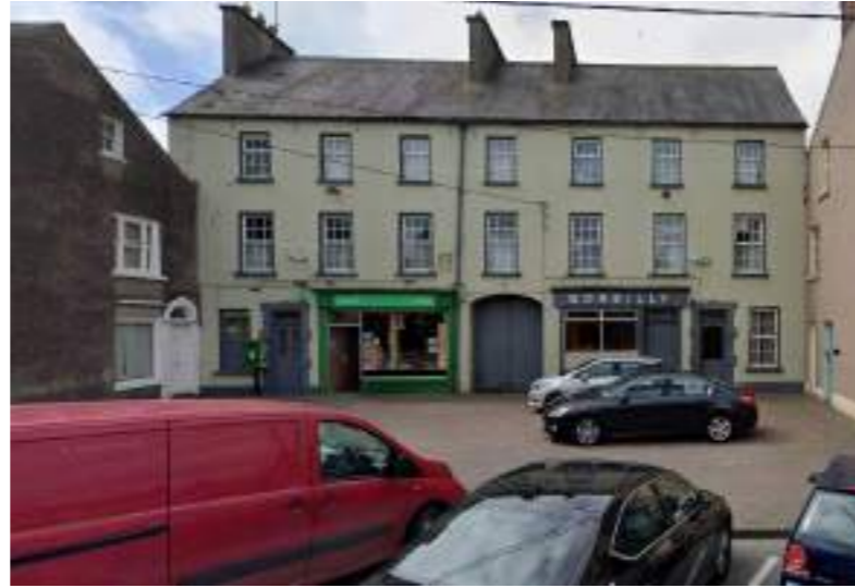
Figure 71 - Bailieborough Main Street - Before Painting Scheme
