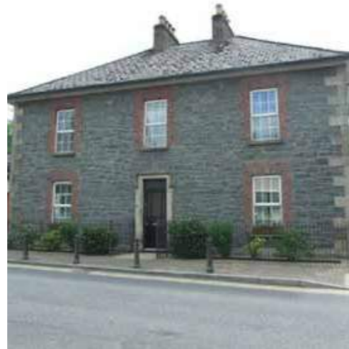
22. House at Barrack St.
