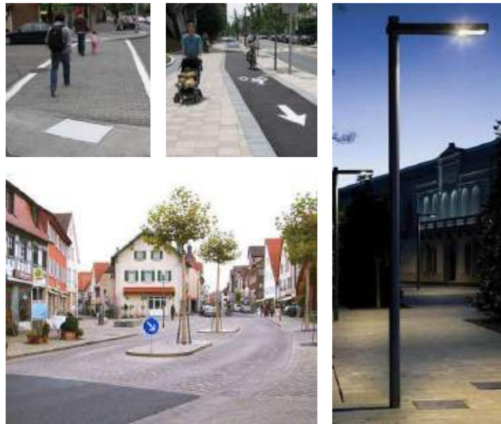
TL: Use of differentiated paving to strengthen the visibility of the crossing TM: Cycle physically separated from traffic on the main street BL: Shared surface R: Example of context sensitive lighting solution
