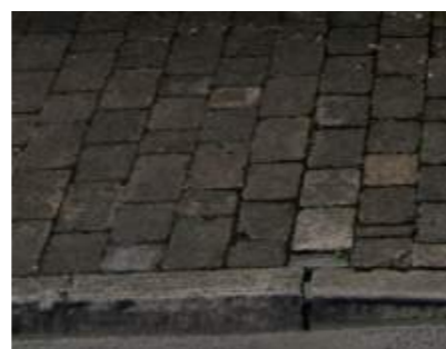
Figure 92 - Pavement at Henry Street
