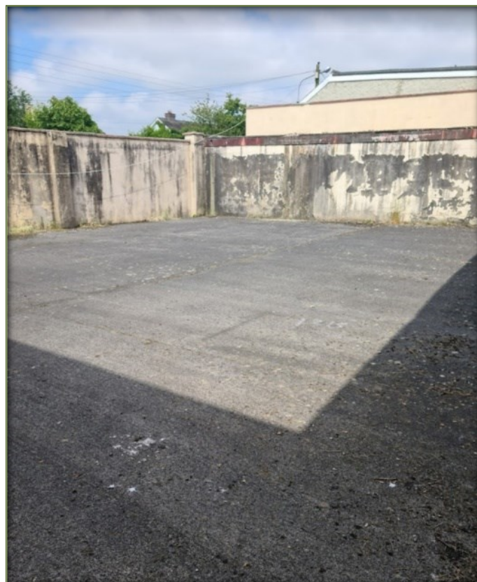
Figure 5b – Photo of Yard
