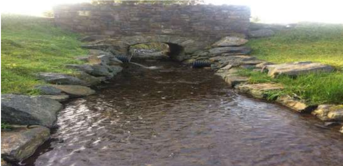
Lackenmore Bridge, Ballyjamesduff – post repair.
