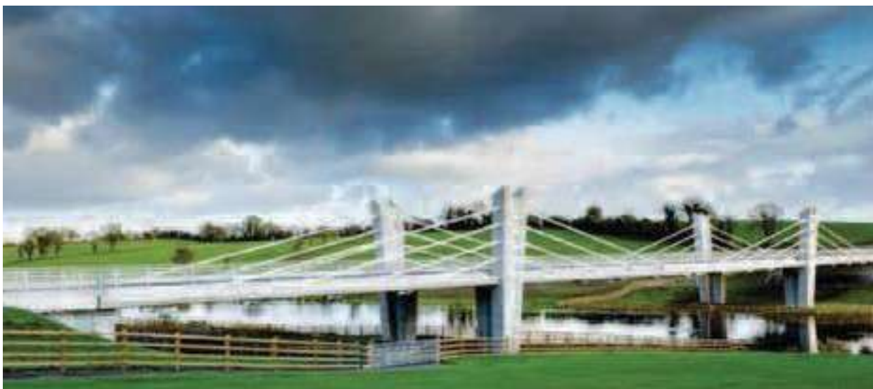
Extradosed Type Bridge over the River Erne
