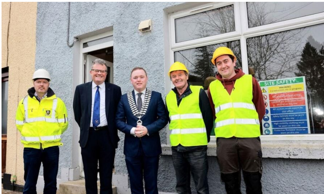
Refurbishment Works in Progress at Jubilee Terrace, Cavan
