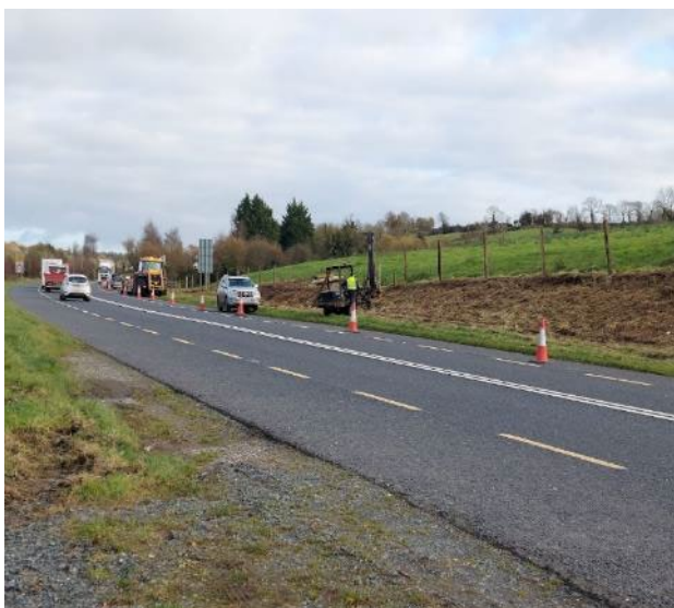
N3 Retro-fencing Works
