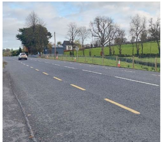
N3 Retro-fencing Works - Completed
