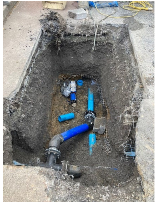
Connection to 100mm UPVC Class C feeding
