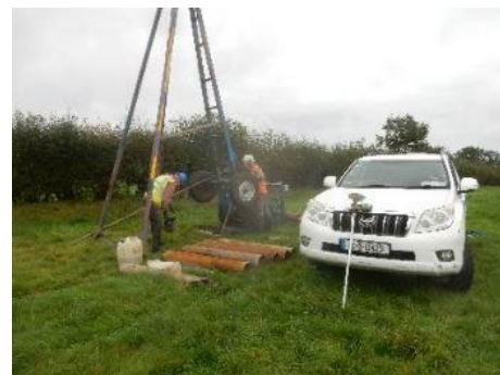
Site Investigation - Coring for soil samples
