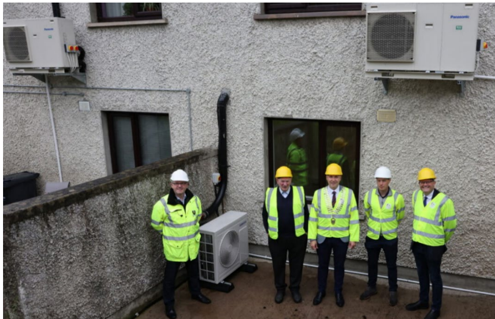
Completed Retrofit Work at Laragh Crescent, Cavan
