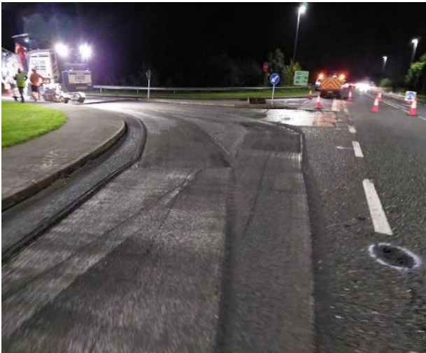
N54/N3 Butlerbridge Junction HD28 Site
