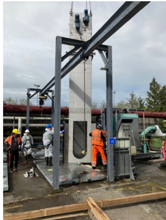
New Screens Being lifted into place.
