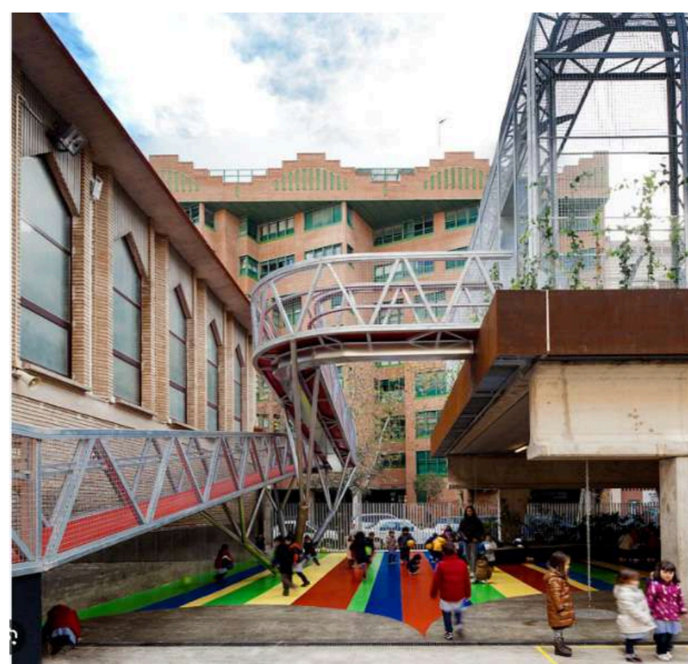
Elevated sports court at Lasalle Franciscanas School by J1 Arquitectos
