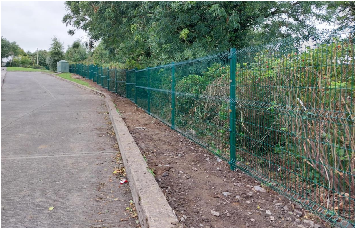
Anti Dumping Preventative works carried out in Ardkeen, Cavan
