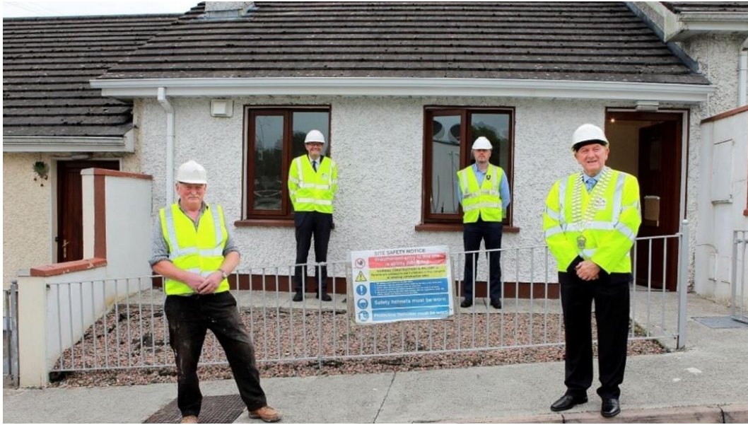
Restoration of a vacant housing unit at Fairgreen Hill, Cavan.
