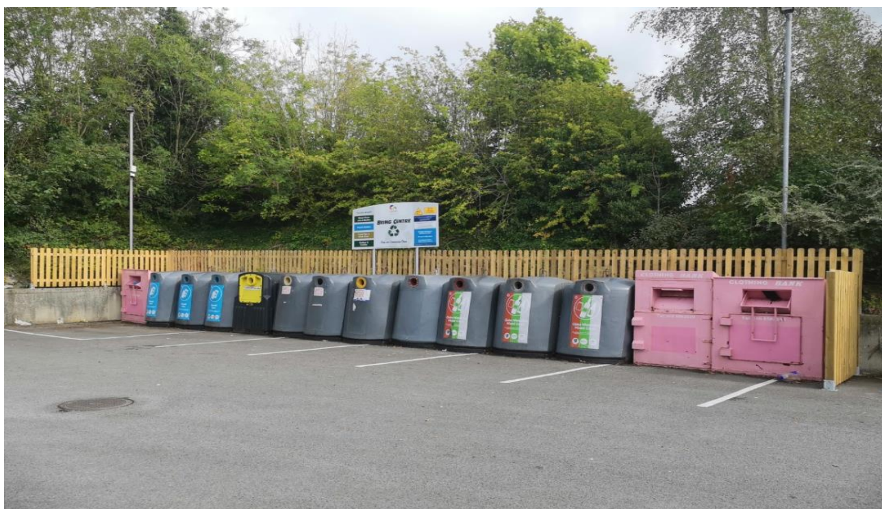
Improvement works at Ballinagh Bring Centre
